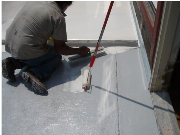
#15 The remainder of the deck where only 60 mils or less is needed may be troweled or rolled into place. ,
