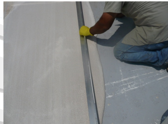
#14 Sand Slurry may be also screeded out by using a flat metal screed. A screw or nail at one end of the screed will help guide the slope to drain.
