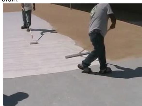
#16 Squeegee and back roll coating. Backroll coating with \frac{1}{2} nap roller. Workman wear spiked shoes for application of coating and back rolling.
