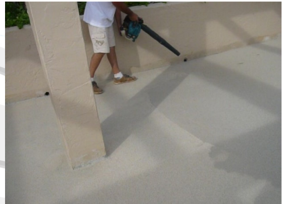
#20 Blow off sand approximately 2 hours or when coating feels completely dry enough to take foot traffic.
