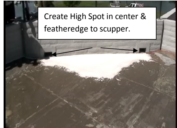
#12 Apply the coating in a triangle manner from the high spot in the center down to a feather edge thin layer at the scupper as shown.
