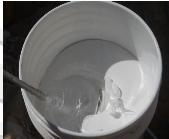
#8 Mix until water and catalyst completely disappears into the coating (about 2 minutes)
