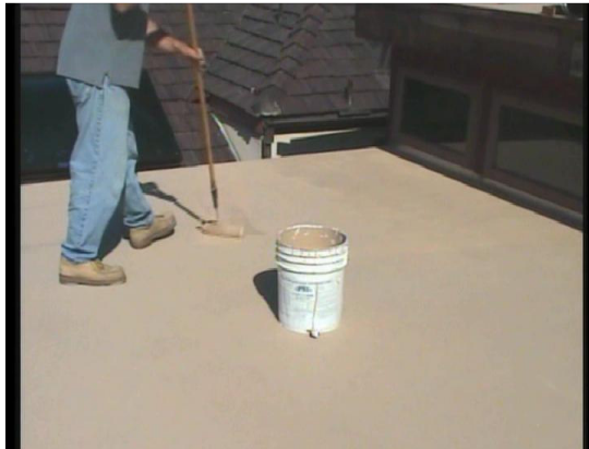
#19 Mix 3 qts of xylene into a five gallon pail of top coat. Apply evenly with a ½"-3/4" nap roller.
