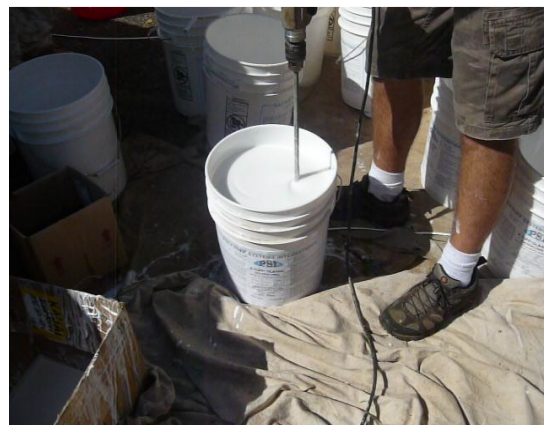
#4 Open on 5 gallon pail and mix from bottom to the top for a minimum of 2 minutes.
