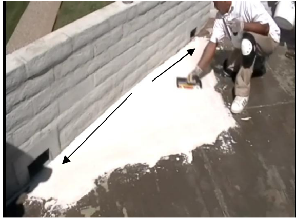
#11 Trowel out coating with a \frac{1}{4} " x \frac{1}{4} " notch trowel or a pool trowel and work from the high spot to the scupper or drain.
