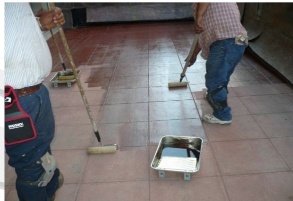
#2 Apply a very thin layer of primer by 3/8" nap roller at 300+ sq/ft per gallon.
