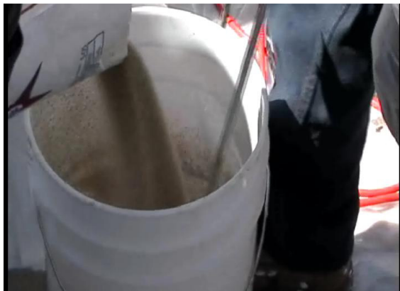
#9 Fill the rest of the pail to the top lip line with 16-30 mesh sand, NO OTHER SAND ACCEPTED. This is the PolyTuff "Sand Slurry" System.
