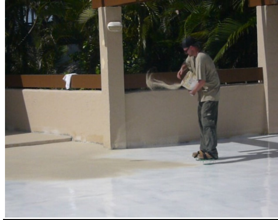
#18 Broadcast 16-40 mesh silica sand to refusal or until the deck looks like a beach.
