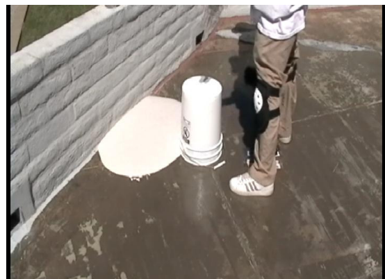
#10 Pour out pail where the coating will need to be the thickest or where you want to make the high spot of the cricket.
