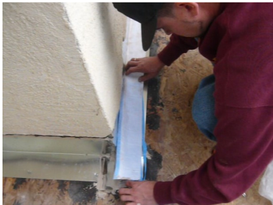
#1 Apply Super Seal Tape to all metal flashings where coating is to be applied. The tape must be completely covered with coating.
