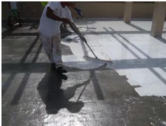
#13 After the cricket is made apply coating by notched squeegee according to the predetermined desired mil thickness.
