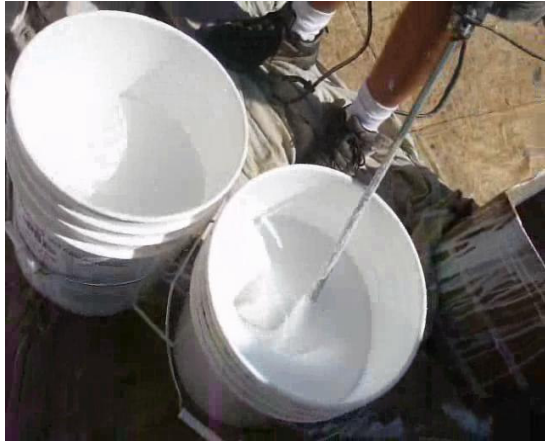
#5 Separate the 5 gallon pail into 2 -2 ½ gallon pails
